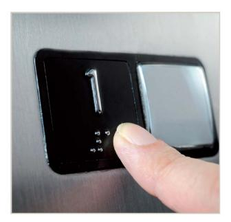
Place tactile elevator floor indicators on the leading edge of the entrance door or landing frame, at a height of 1350mm from the ground.
